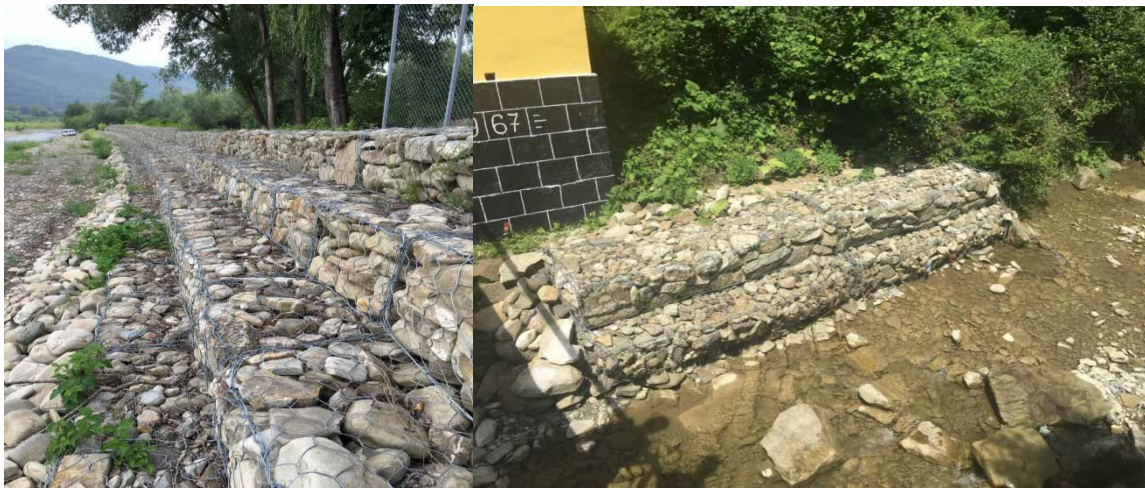
Bank strengthening examples
