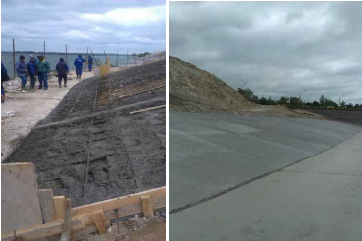
Reinstalling joints between plates
