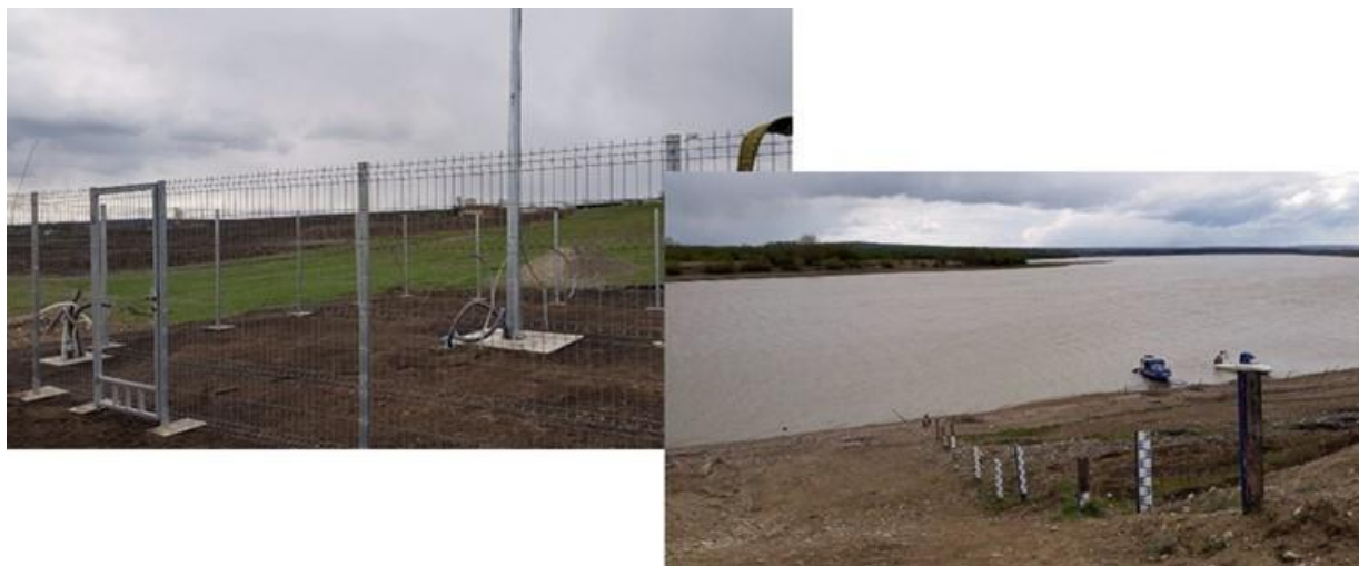
Works stage at Ripiceni automatic station location – april 2016
