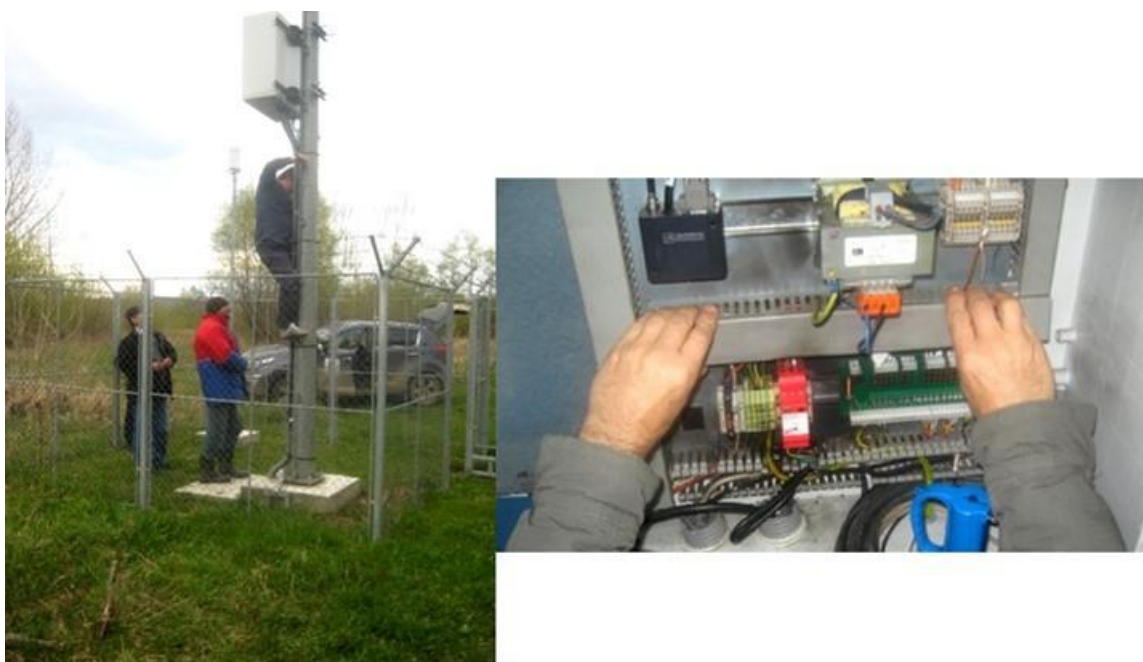
External and internal verification works (Oroftiana and Radauti stations)
