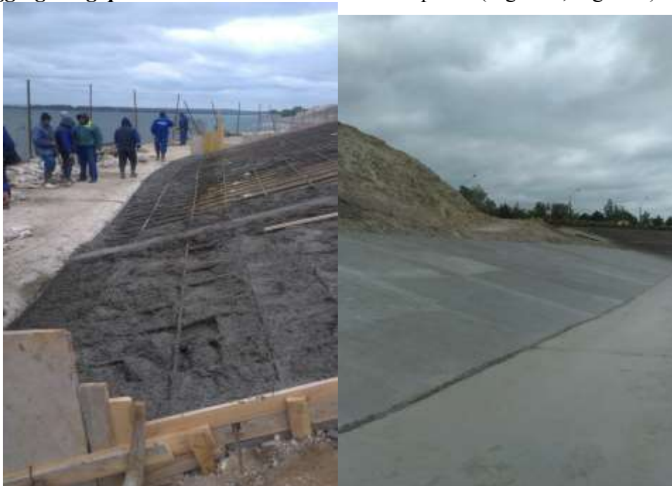
(Figure 2) Reinstalling joints between plates (Figure 3)
